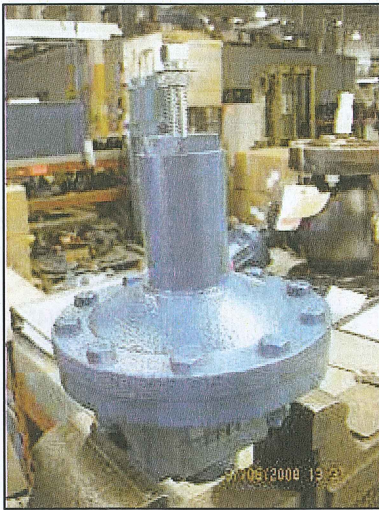
Remove valve from line.
