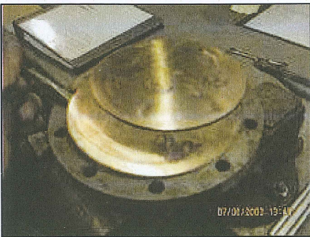
Remove, inspect & clean parts.
